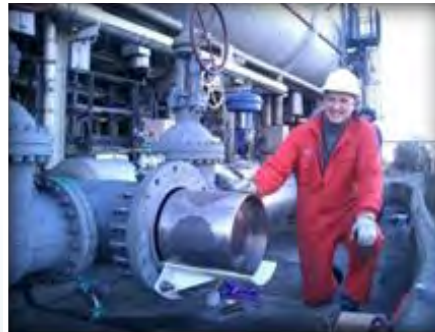
ProSalt (crude desalting)
